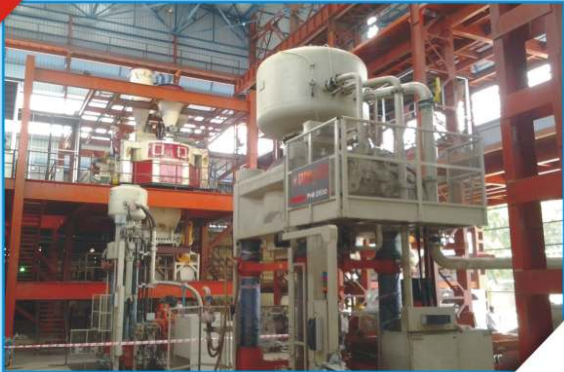
New FCP Plant at Belpahar under Construction
