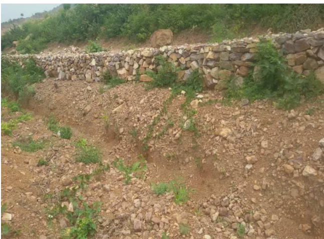
Retaining wall & Garland Drain
